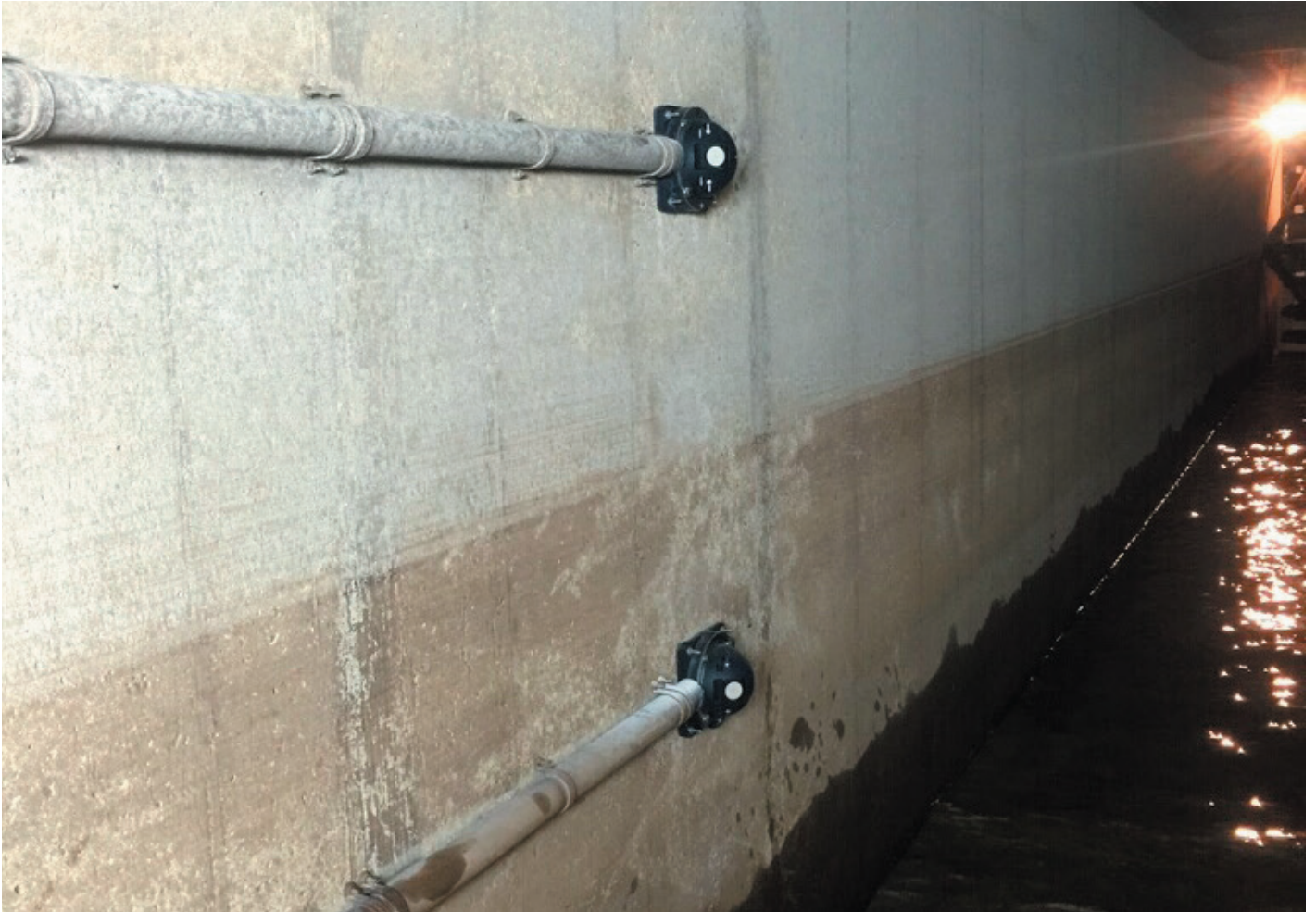
Installation of Kanalis sensors in the Jardine water purification plant
