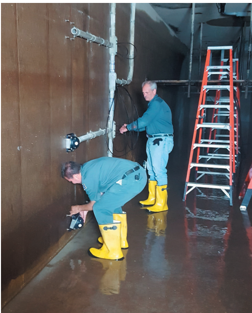
Installation of transducers inside the channel.
