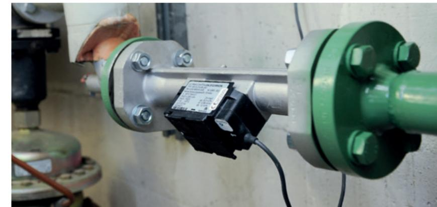
Partie hydraulique DN 25, qp 6,0
